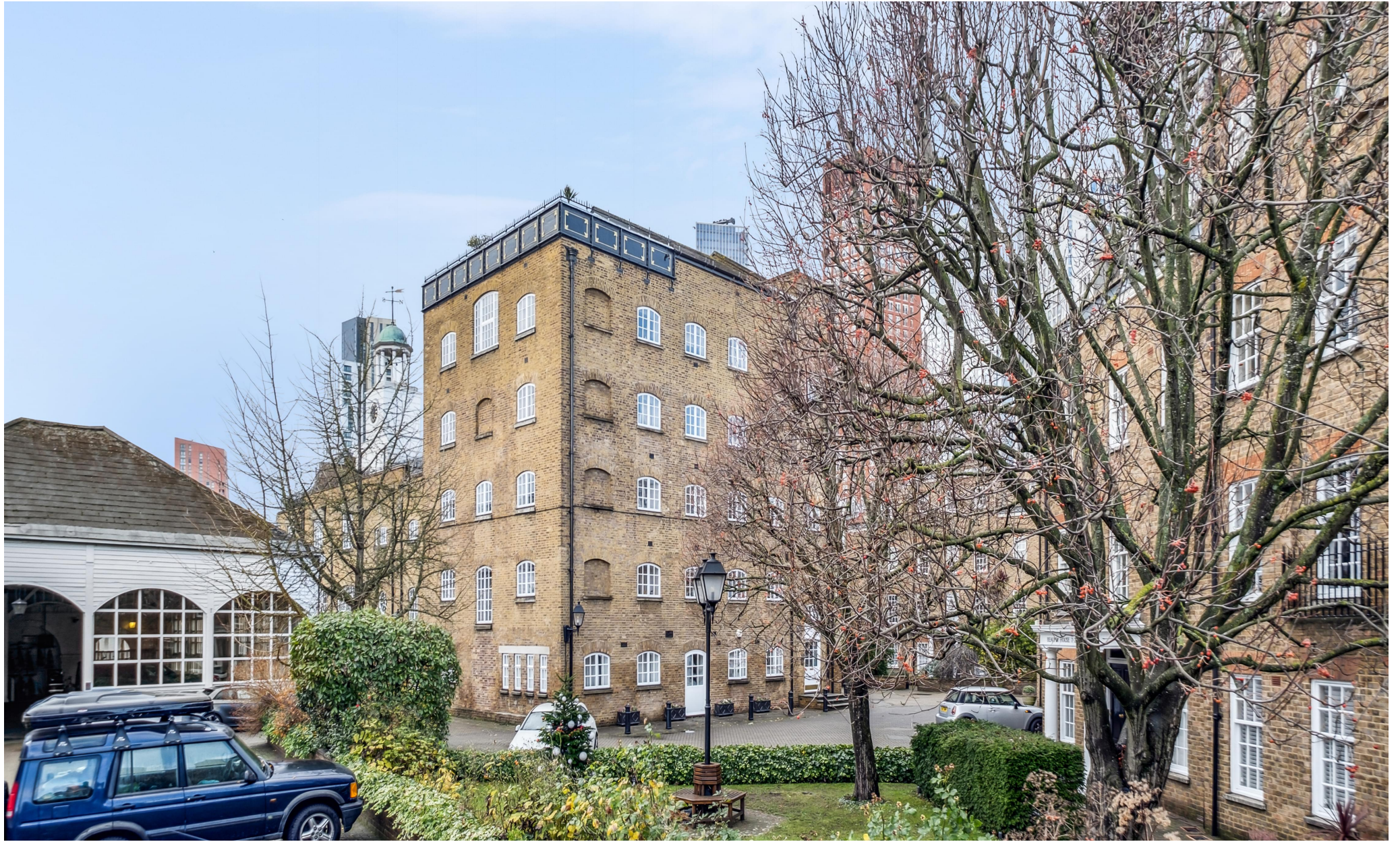
The Vat House, Vauxhall, London SW8
