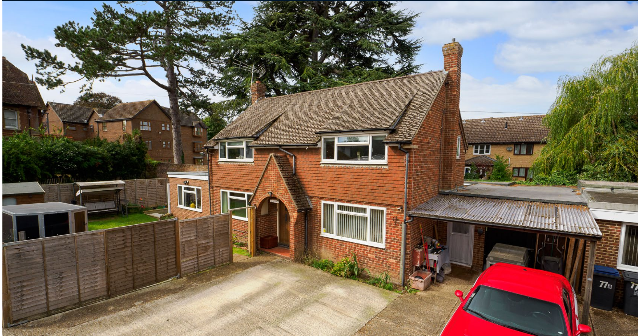
Pippin Cottage, New Dover Road, Canterbury CT1 3DZ
