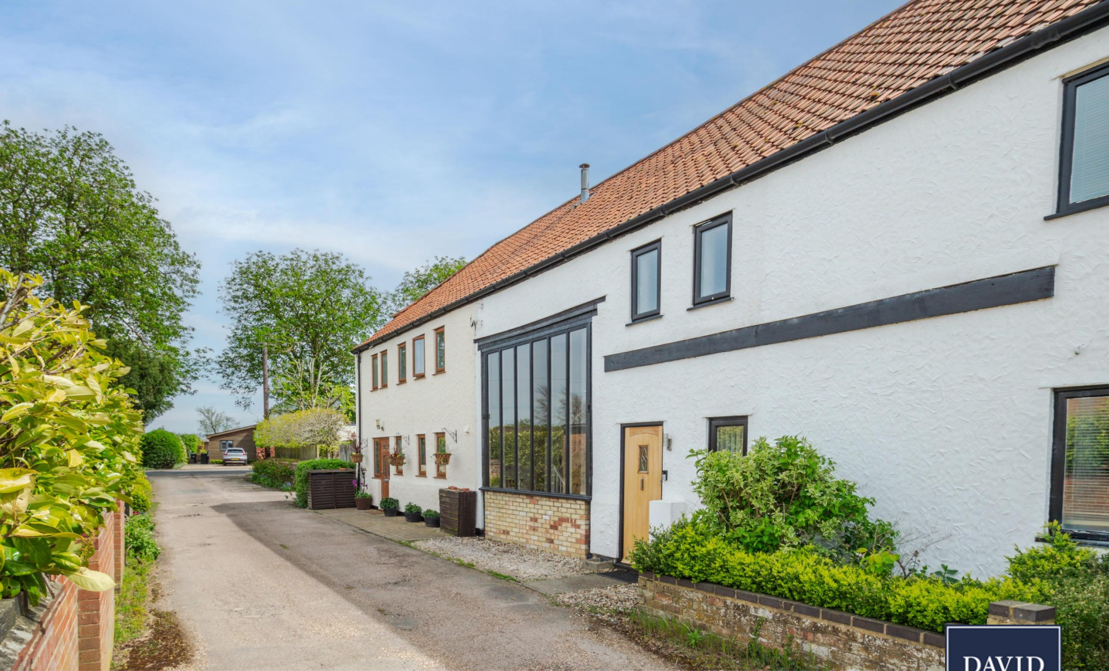
2 Manor Farm Barns, Chippenham
