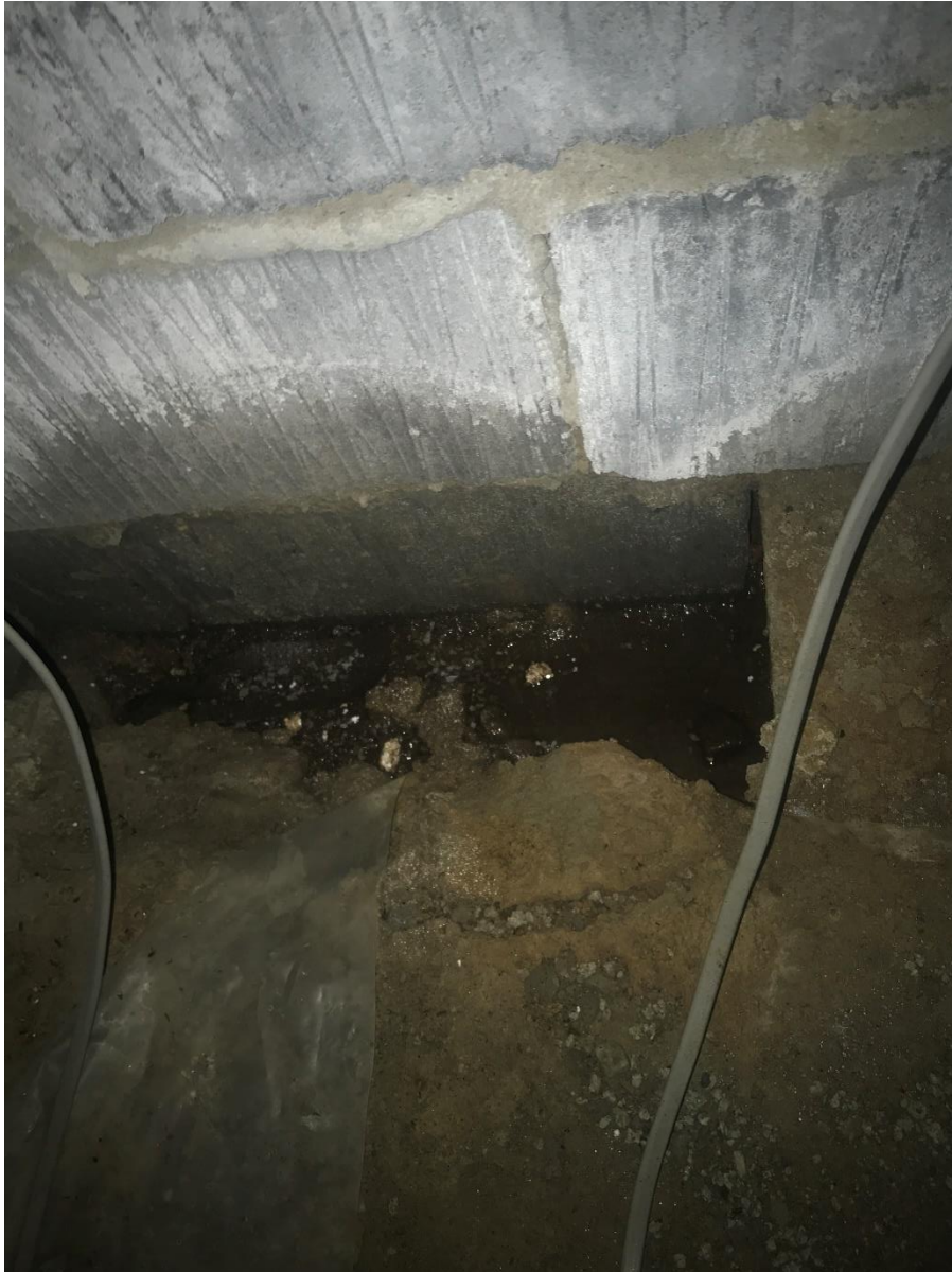
Figure 10 Small void acting as a sump, with a small amount of water noted.
