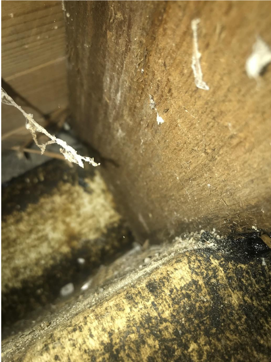
Figure 11 Bearing ends of timber floor joists in good order, with damp proof courses installed below.
