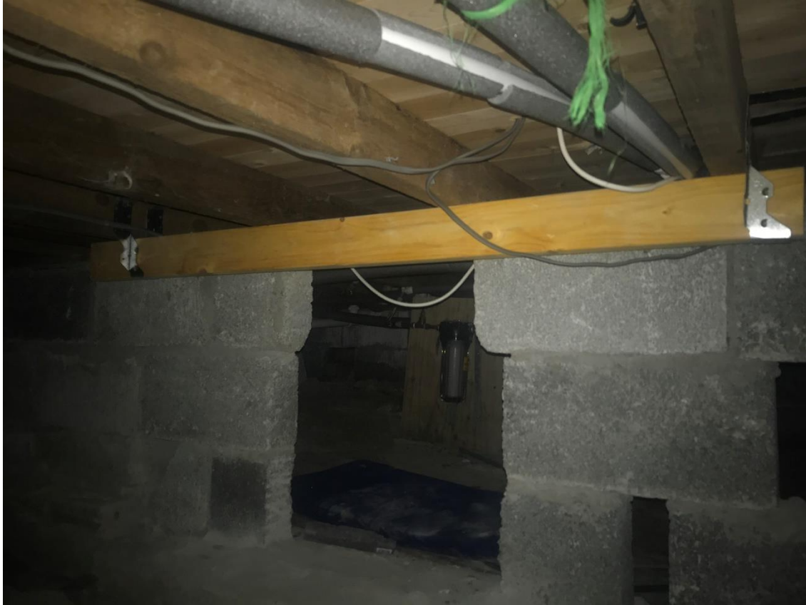
Figure 9 The original sleeper wall did not have concrete lintels installed. Instead, timbers have been used to lintel over. No excessive deflection was noted to the floor structure and this is considered acceptable.
