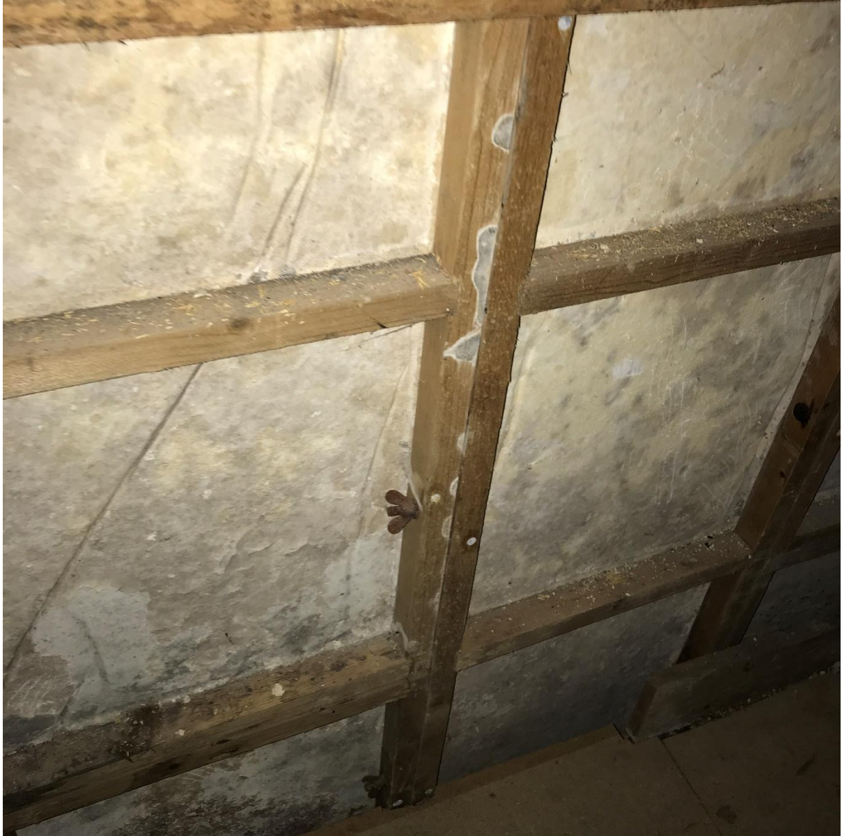
Figure 6 Close up of spandrel panel showing timbers and bolting arrangement.
