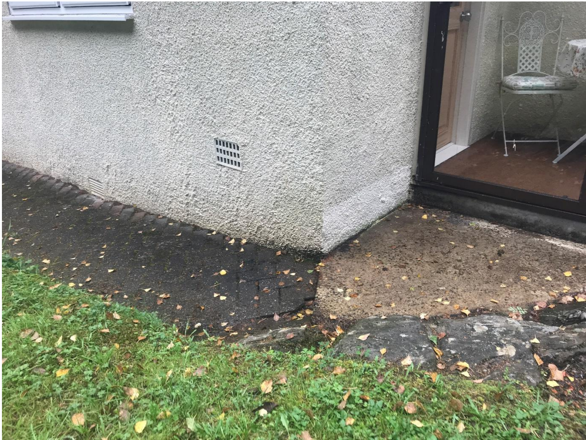
Figure 4 High external ground level at rear. This should be lowered.
