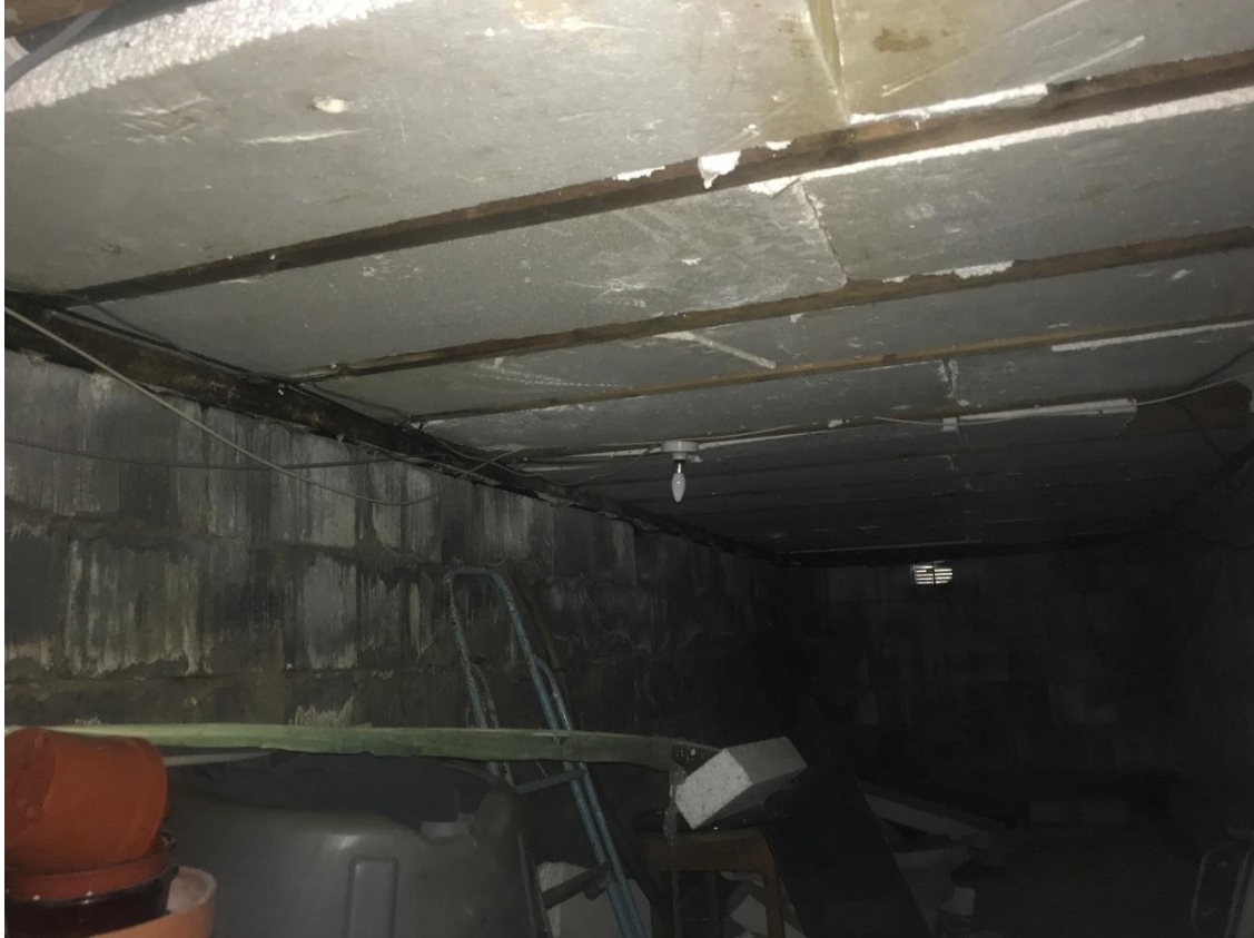
Figure 8 Typical view of floor void, with polystyrene insulation fitted between floor joists.
