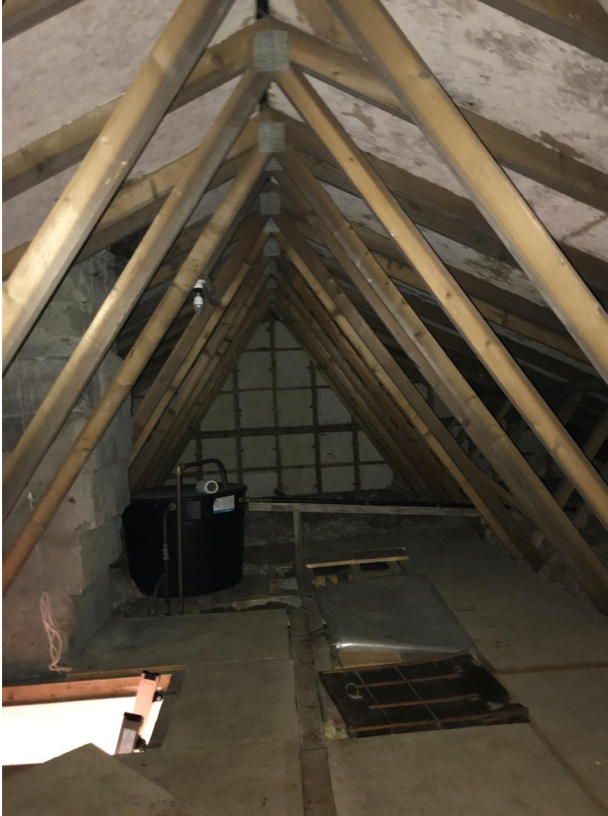
Figure 5 General view of roof void, with fink trusses and exposed gable spandrel panels
