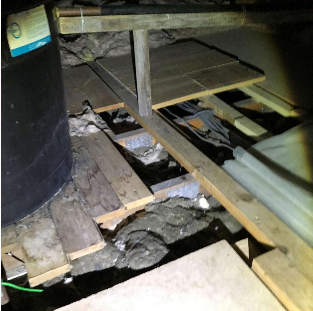
Figure 7 Spliced ceiling joists in acceptable condition.
