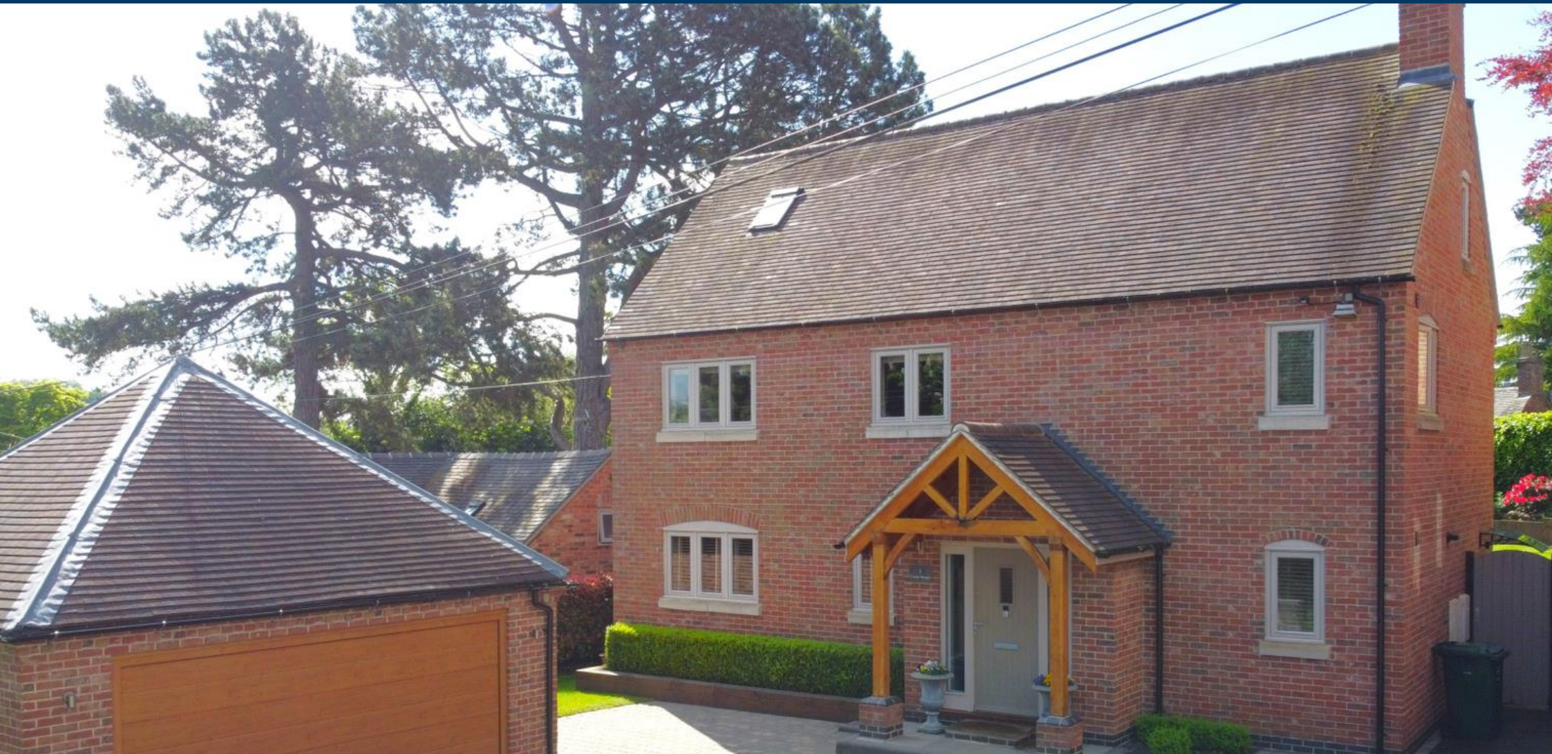
Narrow Lane, Ticknall
