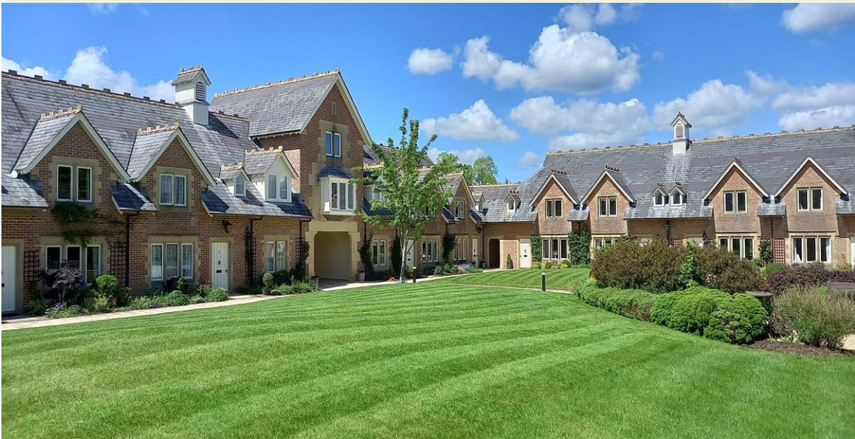
The Courtyard at Walpole Court
