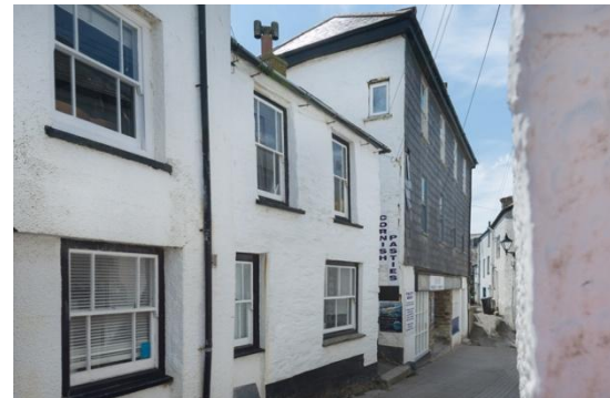
External of Stanley House with its slate hung façade
