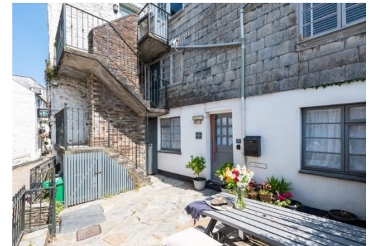
External staircase from The Old Bakehouse
