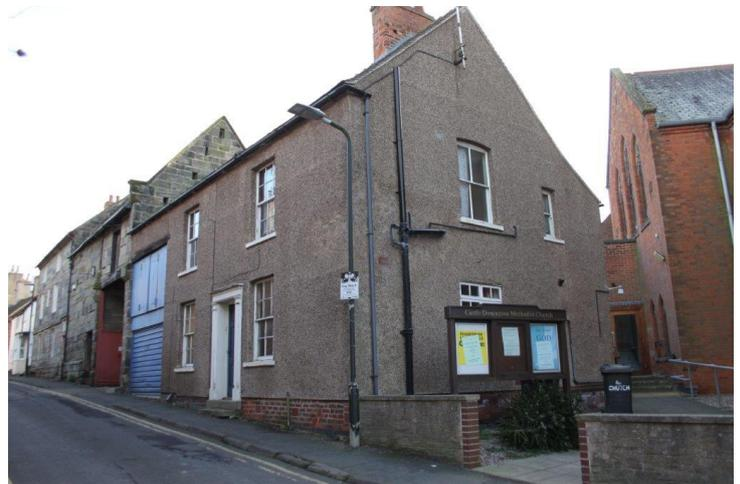
2 Apiary Gate sits to the east of the Church, and is a semi-detached two-storey residential dwelling, and is believed to predate the Church. The building appears to be of traditional solid brick construction with a rendered external finish, under a pitched timber support roof with tile cladding. The building has the benefit of timber single glazed windows, part fitted kitchen and bathroom, and also benefits from an integral garage with loft room over, and enclosed rear yard.
