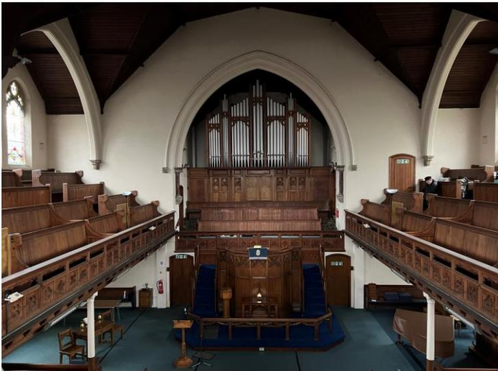
The Chapel has fixed pews, metal-framed stained glass windows to the east and west elevations, underlined timber trussed roof with spot lighting, and electric heating. The area benefits from a balcony to the perimeter, which is of hardwood construction on cast-iron supports, with fitted pews. To the rear of the Altar is a Choir Stand, and Organ.
