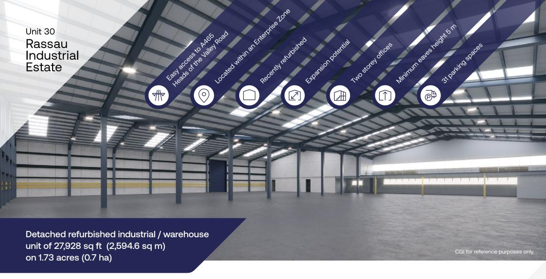
Unit 30 is a detached two bay industrial / warehouse unit of steel frame construction. Elevations are part brick and plastic coated steel sheeting. The roof has similar sheeting incorporating translucent roof lights. There is a two storey office / amenity block to the front elevation.
