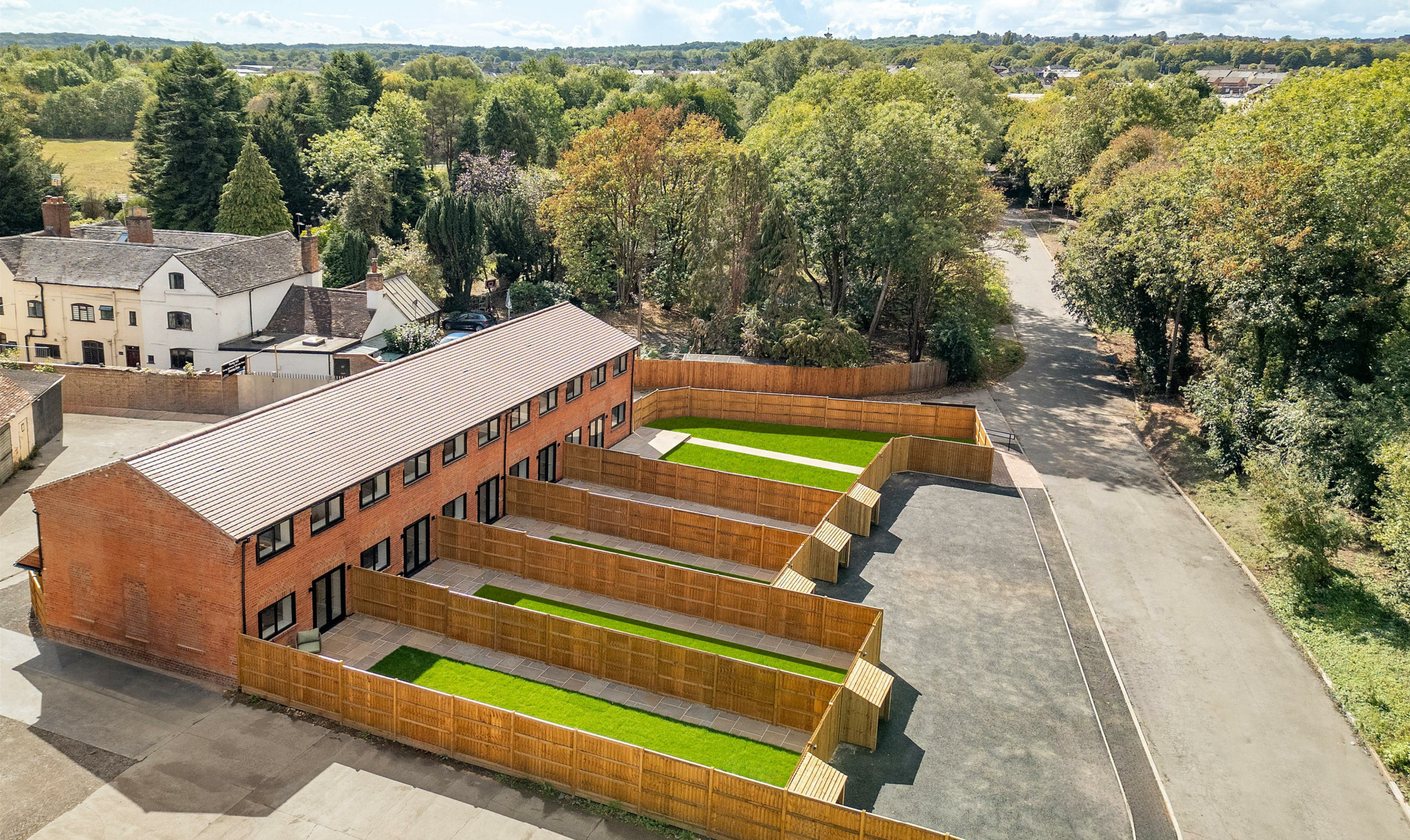
Mill Cottages , Marlfield Lane Redditch, B98 8PU
