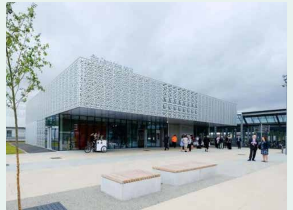
Cambridge North Train Station
