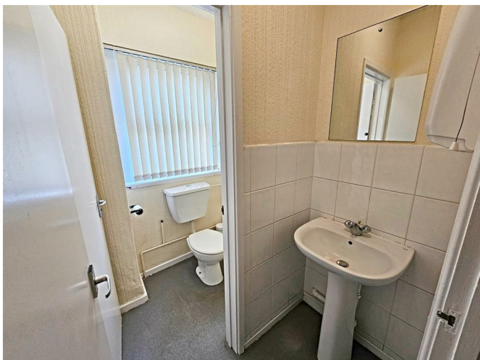
WC, wash hand basin, part tiled walls, extractor fan.
