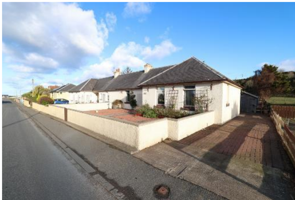
Below: Front of Property
