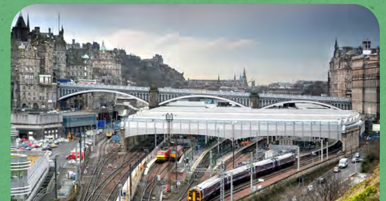
GREAT TRANSPORT LINKS INCLUDING ACCESS TO TRAM, BUSES AND TRAIN STATIONS
