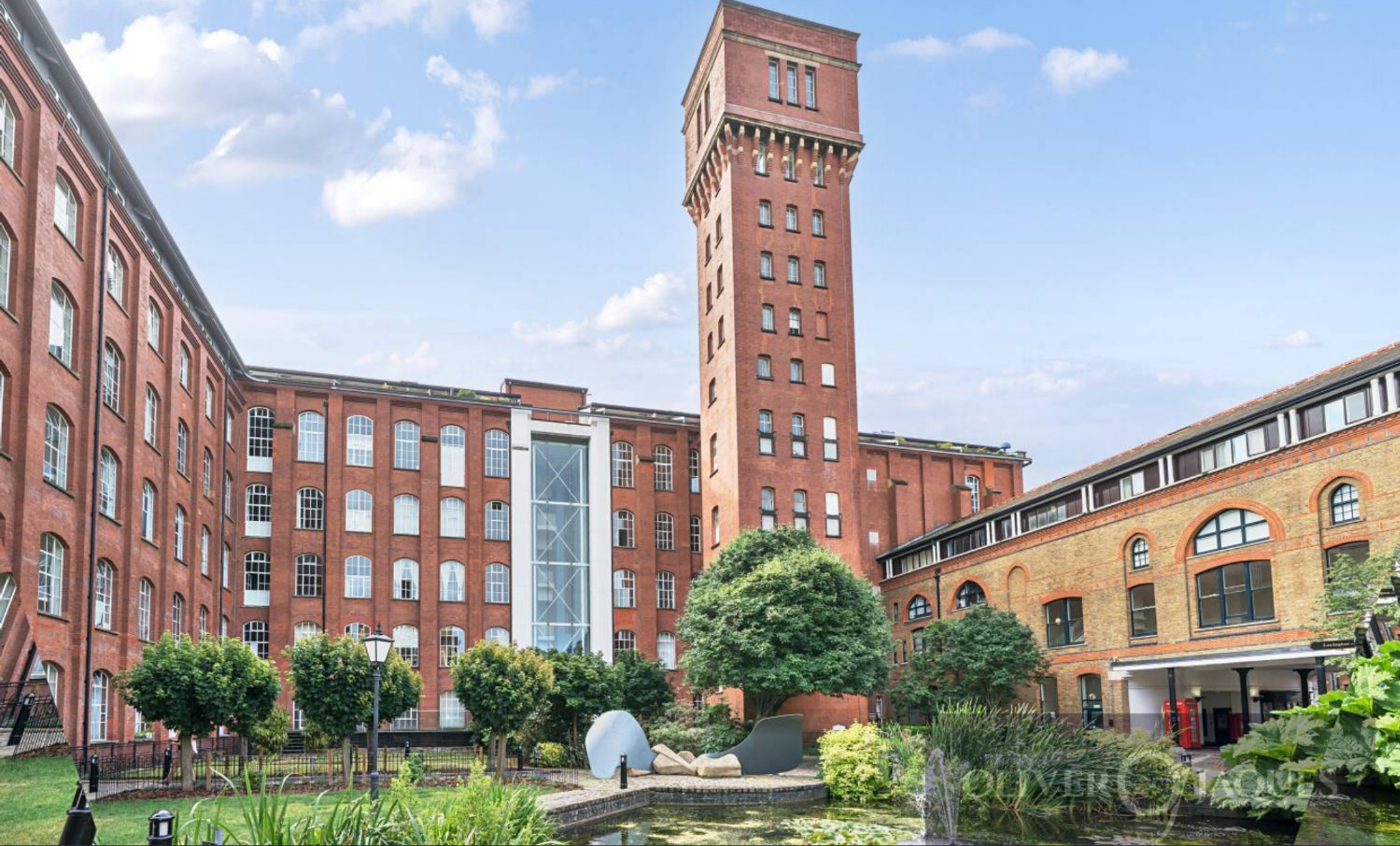
Lexington Building, Bow Quarter, 60 Fairfield Road London
