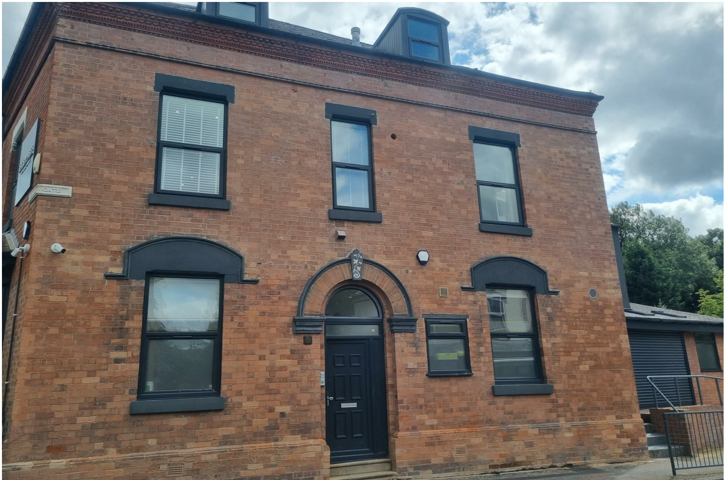
Flat 2, St George`s Apartments, 119 School Road, Moseley, Birmingham, B13 9TX
