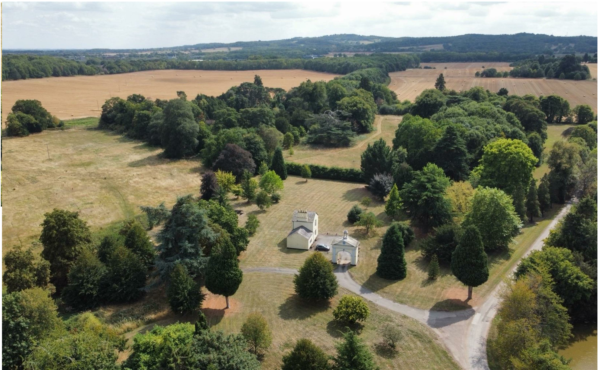
The Shooting Lodge Garendon Park Estate, Loughborough, Leicestershire, LE11 4SH
