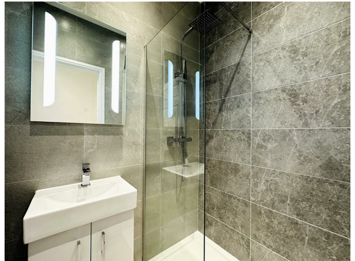
Walk-in shower cubicle with chrome trimmed shower screen, chrome shower and further fixed head shower. White wash hand basin with chrome mixer tap over set into white high gloss vanity unit with chrome handles. The room is tiled on all walls to ceiling height as well as floor. Illuminated mirror, extractor fan and chrome heated towel rail.
