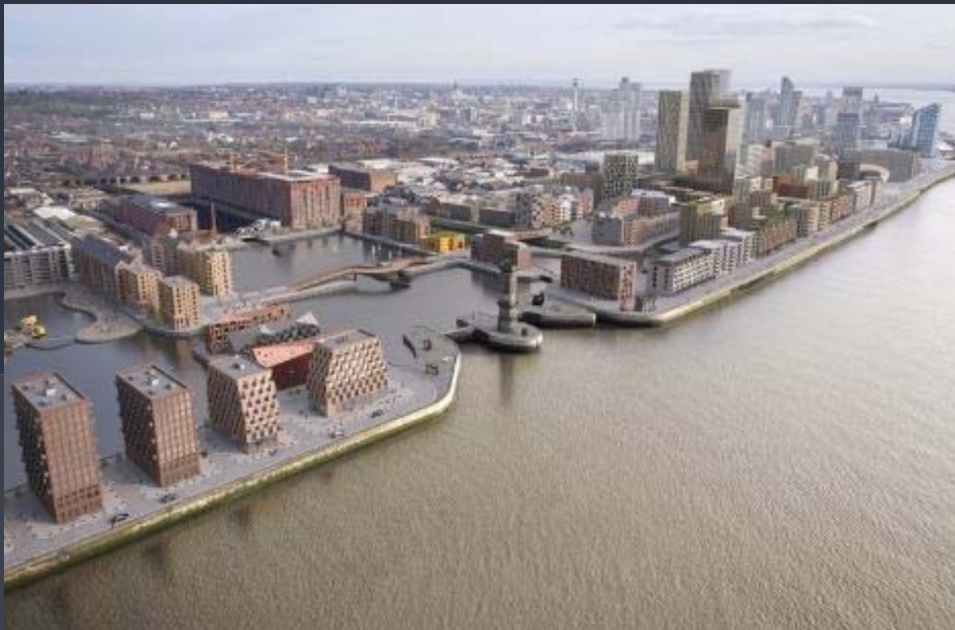
FORMER IBS BUILDING, LIVERPOOL
