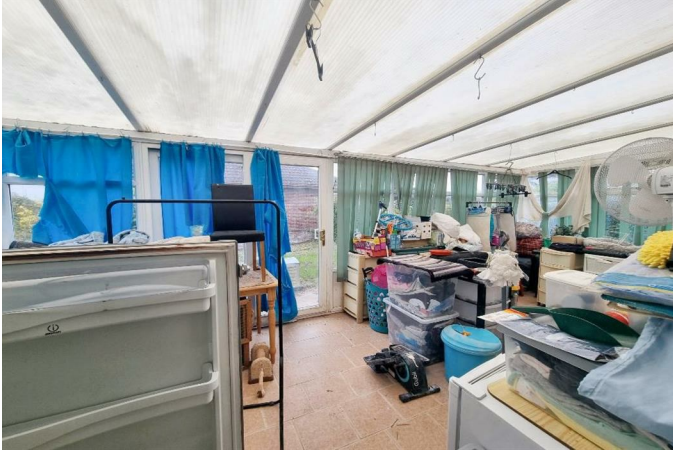
PVCu double glazed construction with polycarbonate roof.
