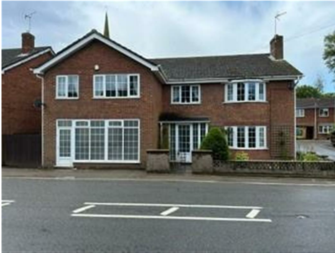
PVCu double glazed window to side.
