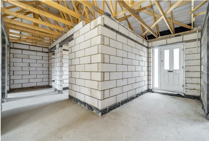
Entrance door to front aspect. Airing cupboard.
