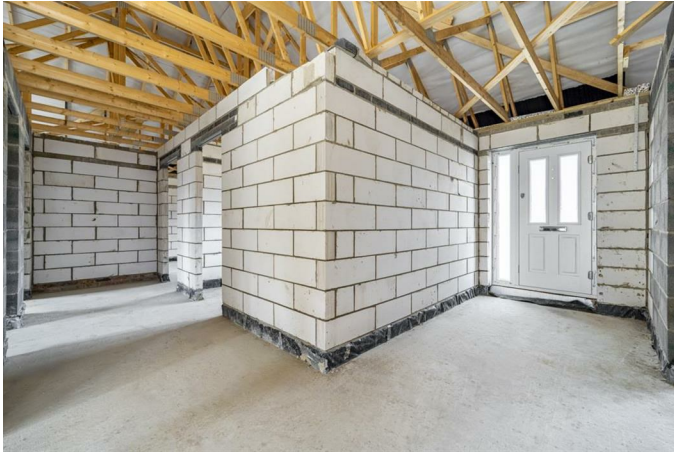
Entrance door to front aspect. Airing cupboard.
