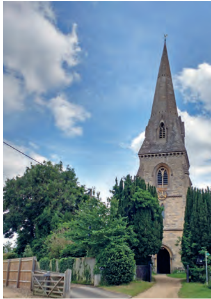
St. Michael's church, Steeple Claydon
