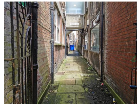
Access from Victoria Arcade
