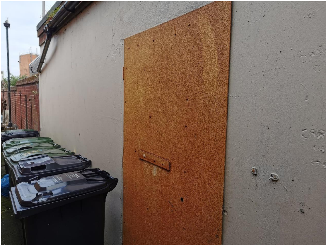
South Side Entrance
