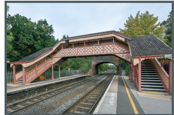
Hagley Train Station
