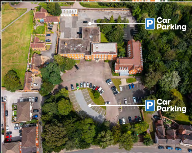
Car park constructed using environmentally friendly and sustainable methods and materials.
