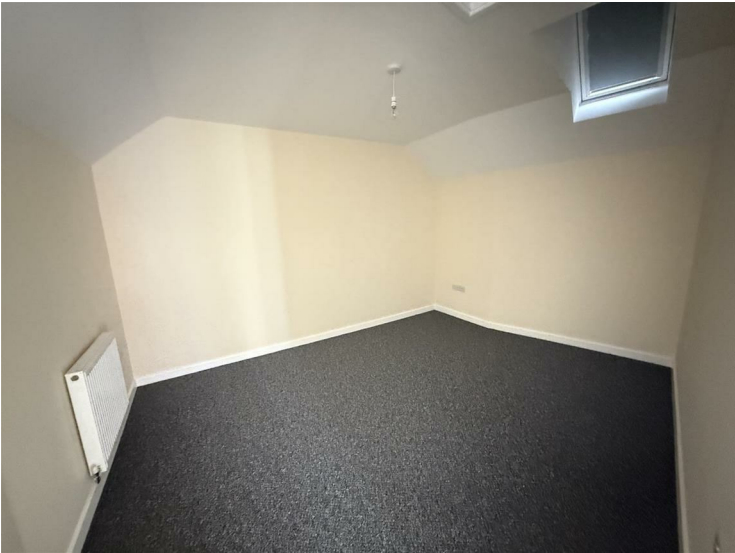
Velux roof window, radiator.
