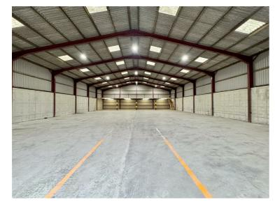
A large single span portal frame building being approx 20' to eaves to allow for larger equipment,
