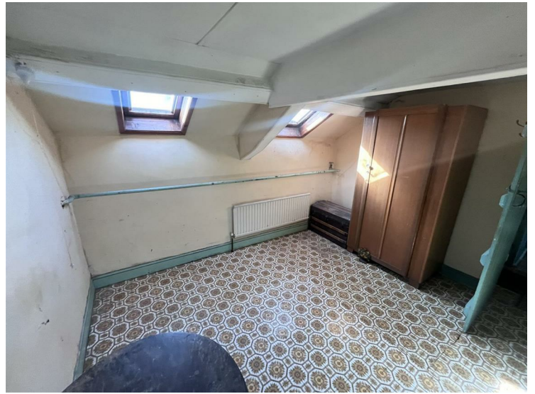
Radiator, 2 sky lights, front window
