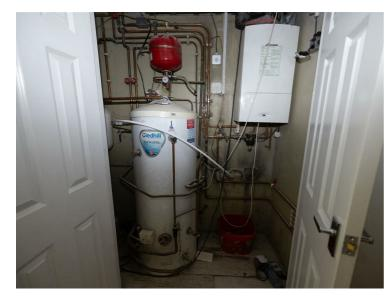
Worcester Bosch Greenstar lpg fed system condensing boiler with pressurisation unit feeding hot water and central heating Fully tiled, Aqualisa push button power shower, toilet and wash to the majority of the house.
