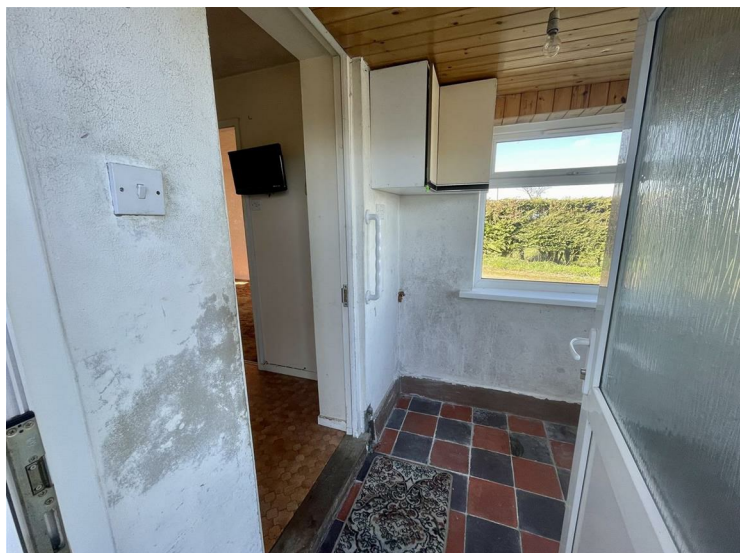
Side entrance door.
