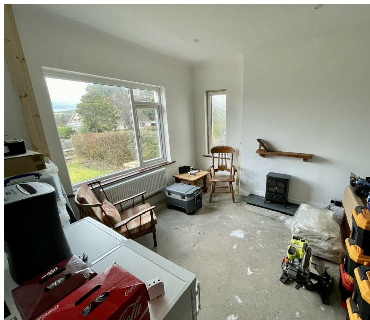
Electric stove with slate hearth
