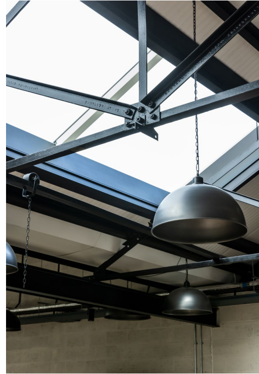
Refurbished Steel Beams
