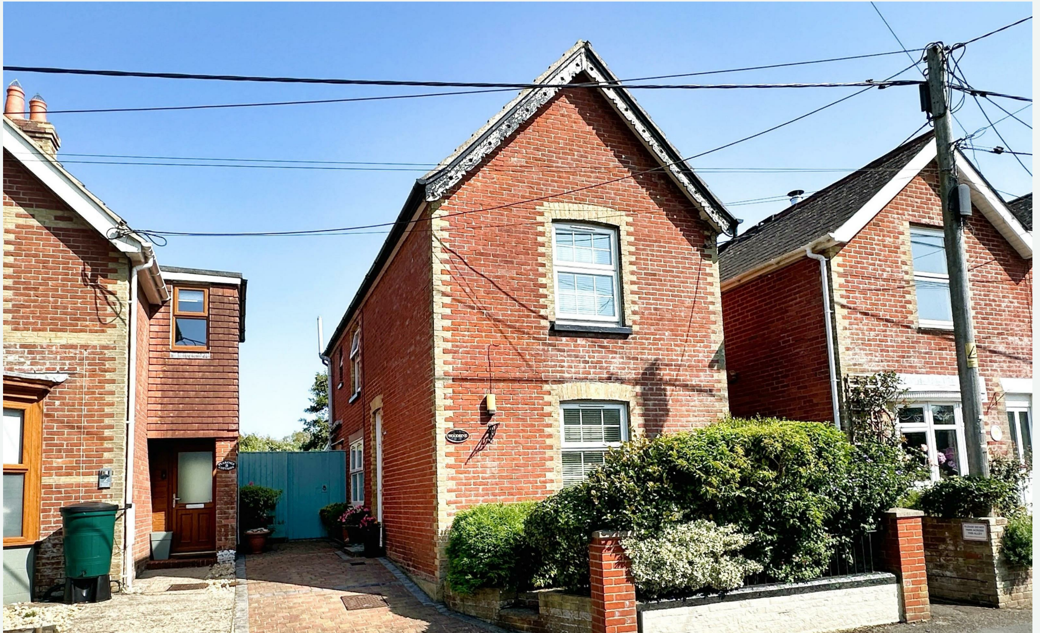
Woodbine Cottage, Queens Road, Freshwater, Isle of Wight
