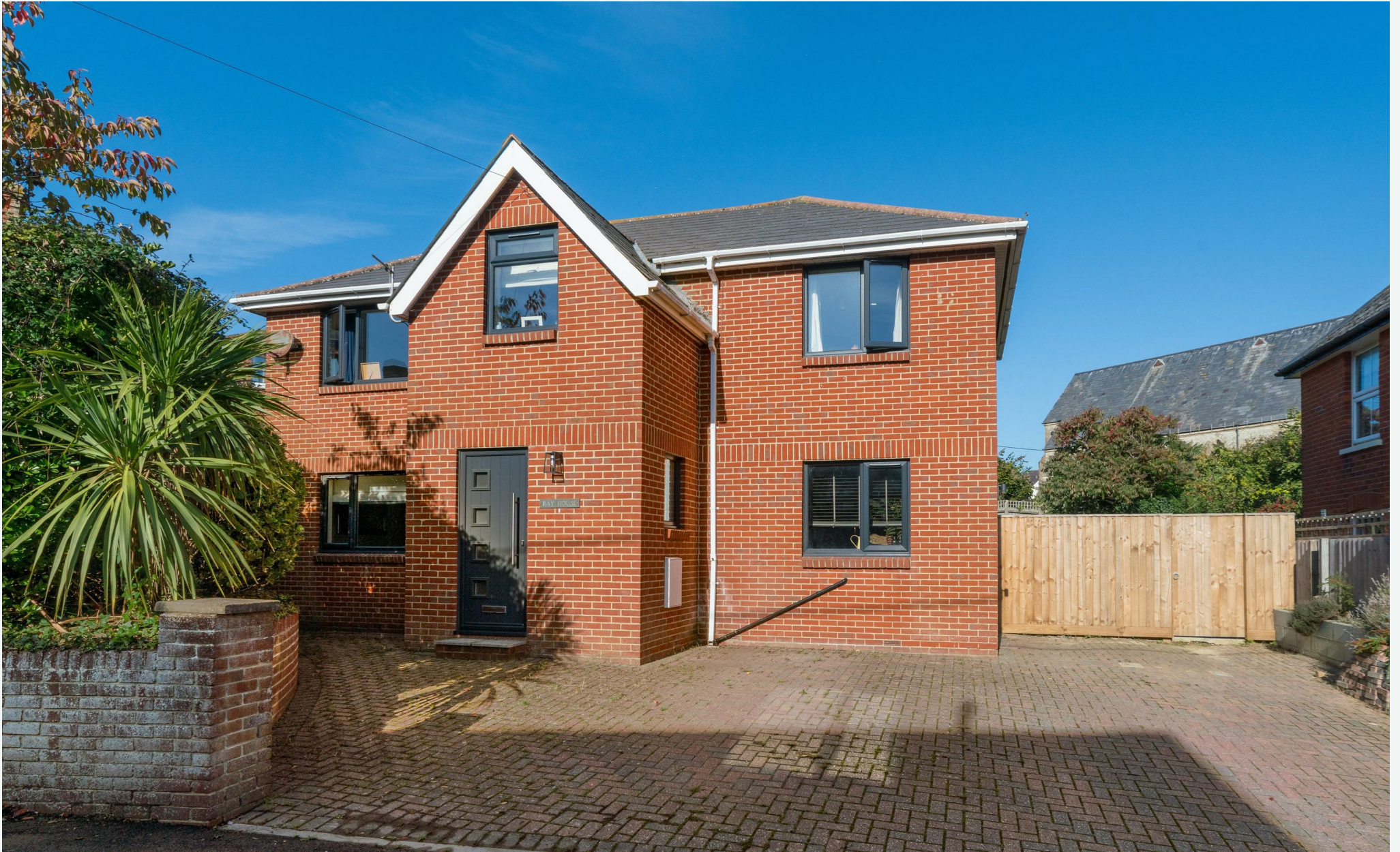
Bay House, Blackbridge Road, Freshwater Bay, Isle of Wight
