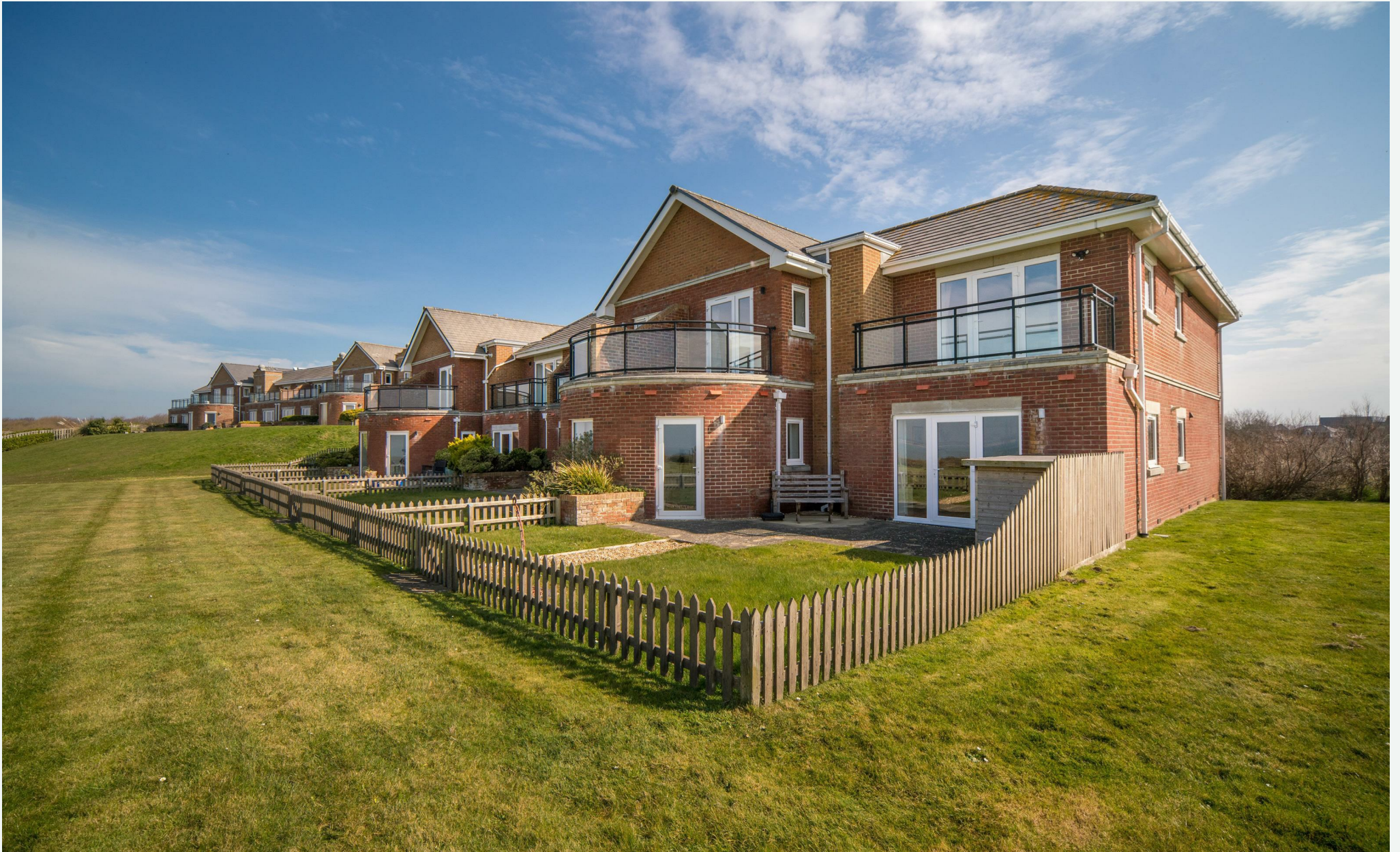
1 Battery Court, Hurst Point View, Totland Bay, Isle of Wight
