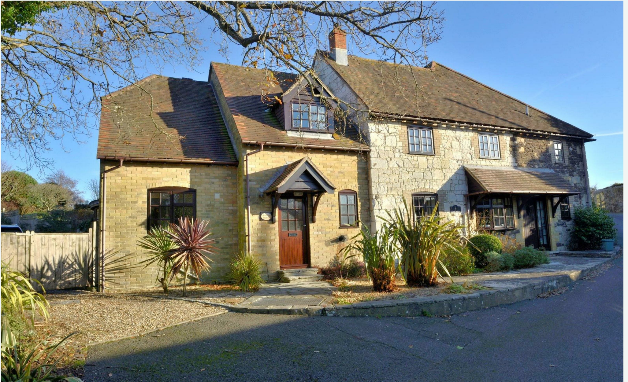
Millers Cottage, Mill Lane, Brighstone, Isle of Wight
