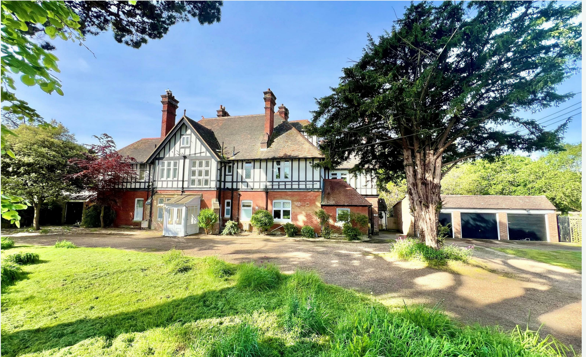
3 Afton Lodge, Afton Road, Freshwater Bay, Isle of Wight
