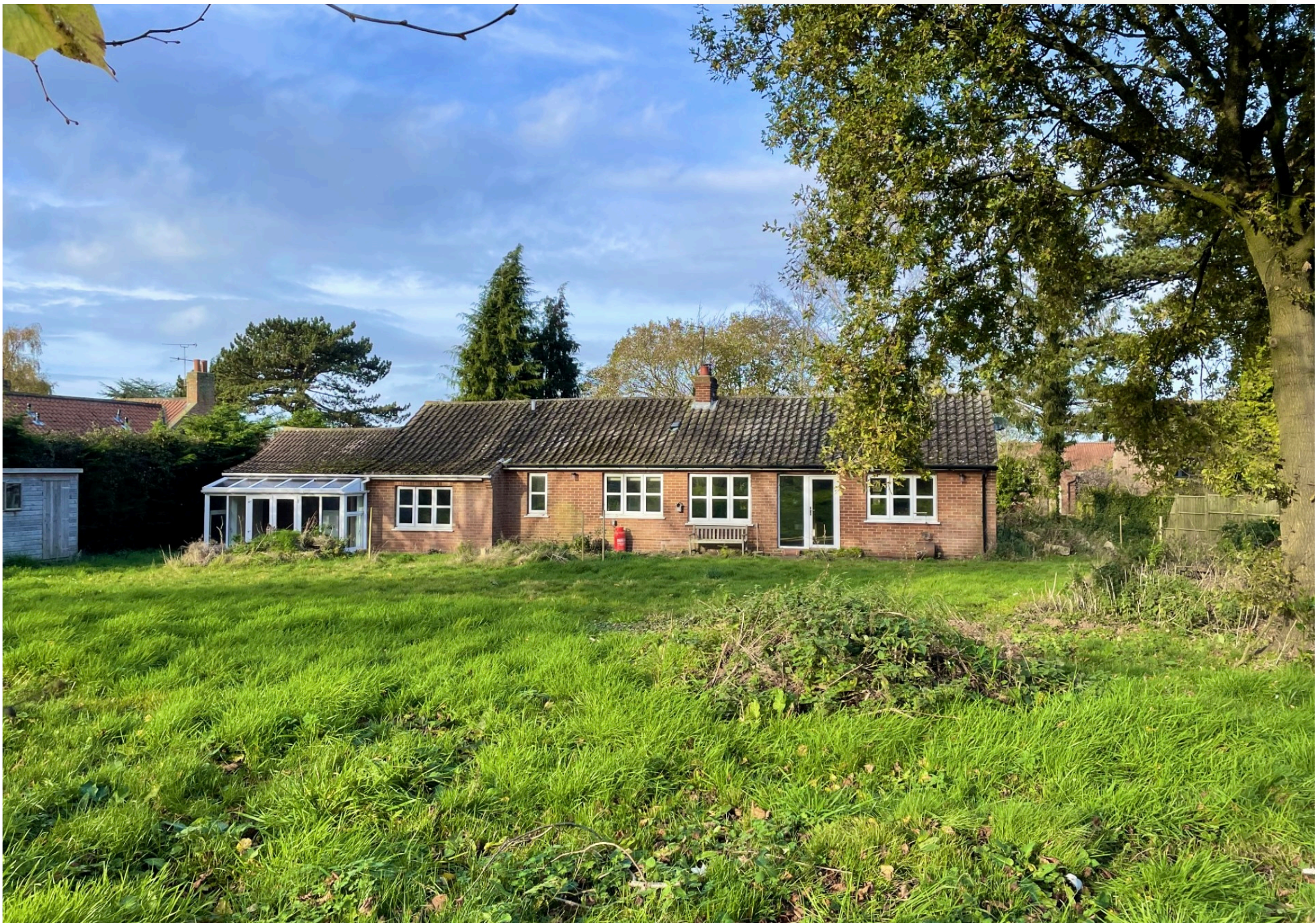
Existing building: 3 beds, 2 baths, and 1 reception room.
