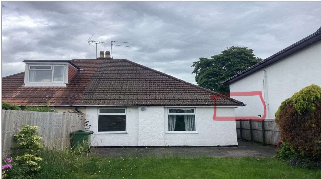
Check roof tiles
