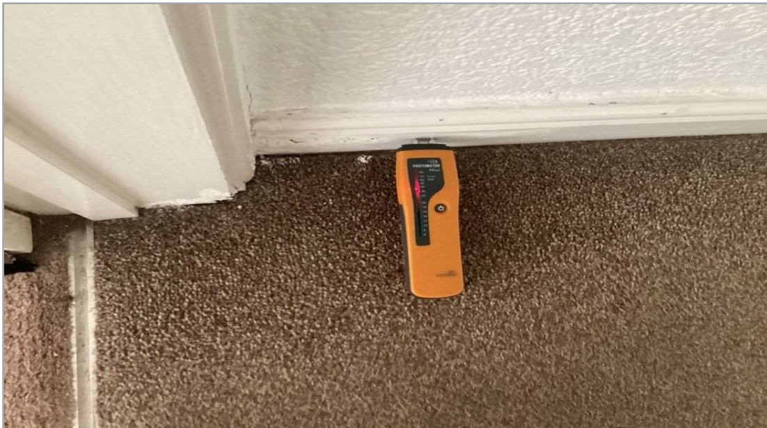
Opposite side of bathroom wall
