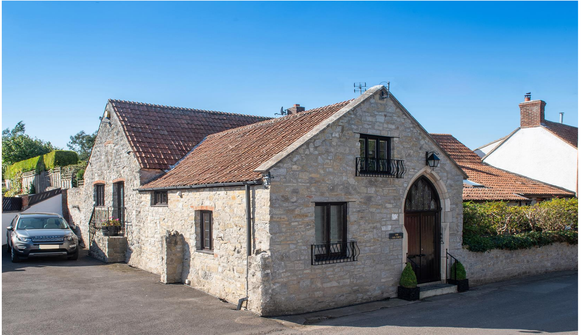
The Old Forge, Stawell
