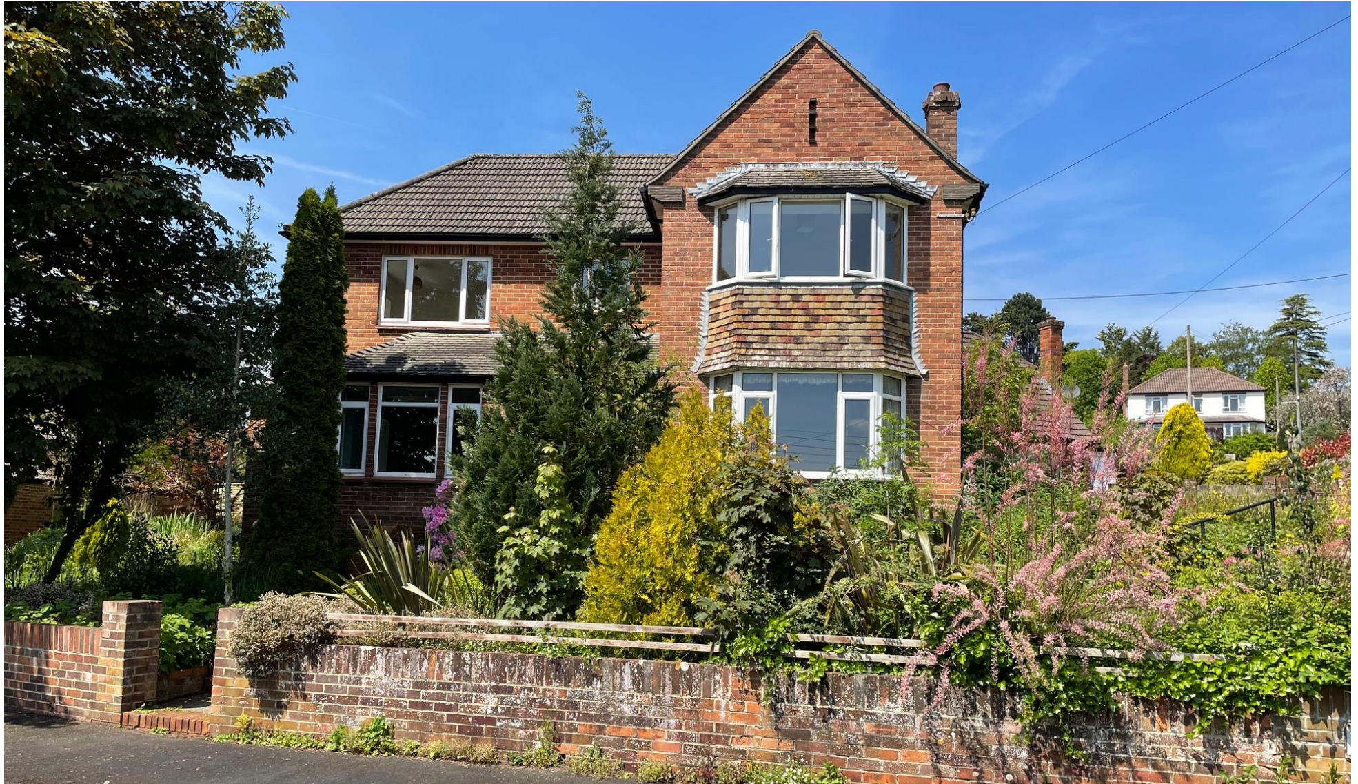
3 Fir Tor Avenue, Wells
