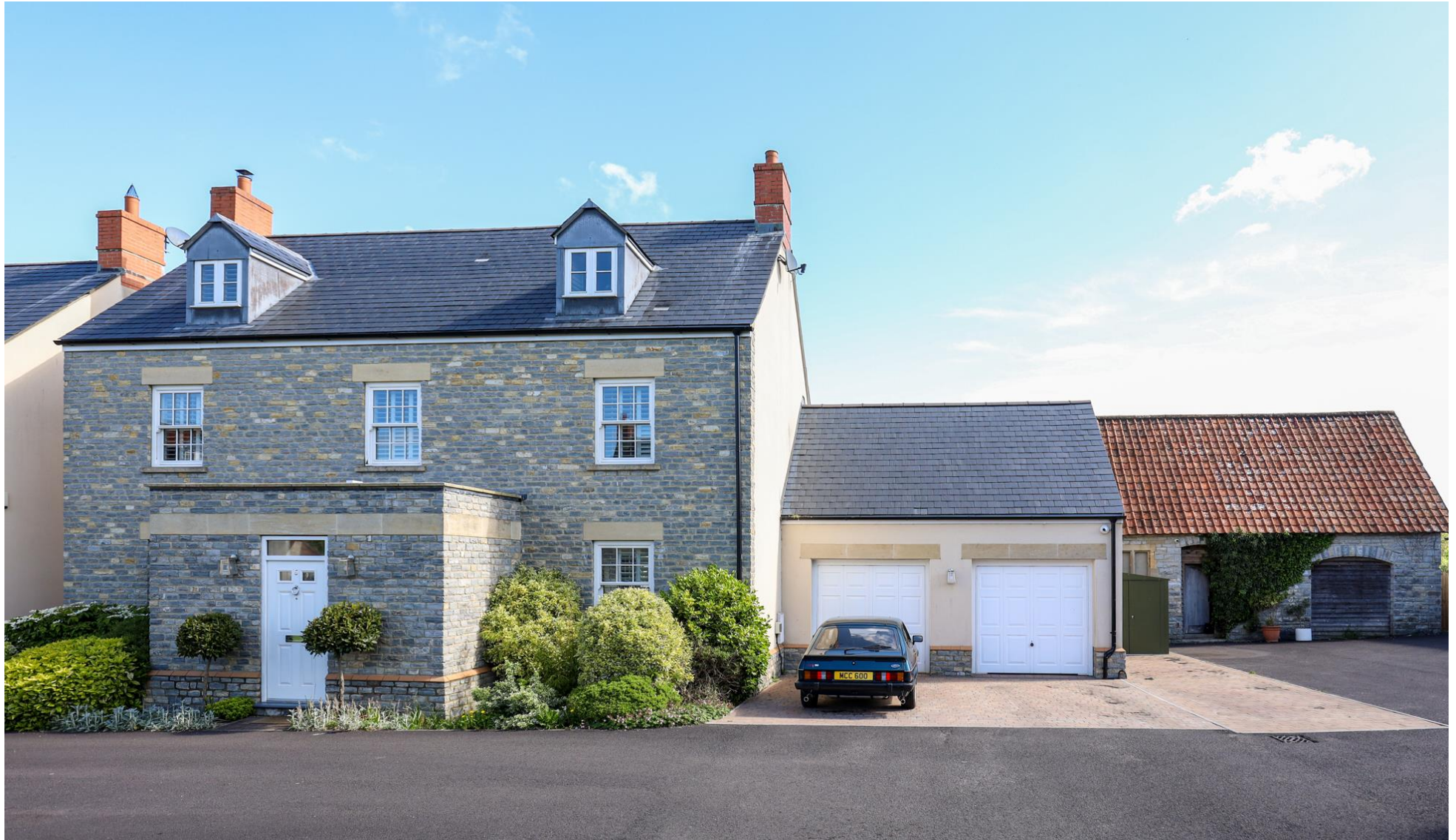
5 Grenville Court, Butleigh
