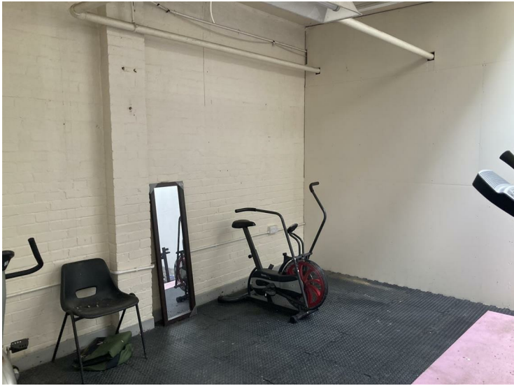
Painted brick walls with partition walls and roof lights.
