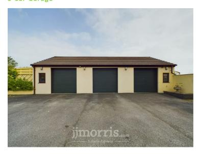
Of cavity concrete block construction with rendered and coloured elevations under a pitched concrete tile roof.
