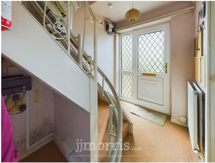
Stairs rising off to the first floor, under stairs space, fuse box, radiator, door to:-
