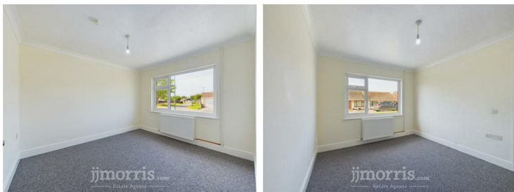
Upvc window, radiator, covered ceiling.
