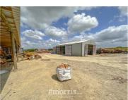
The main building is of a steel portal frame construction, externally clad with profile steel sheeting, with doors to the front and side. The minimum internal eaves heigh its approximately 4.5m.
